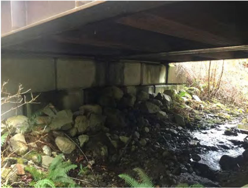
Right Bank Abutment when facing downstream
