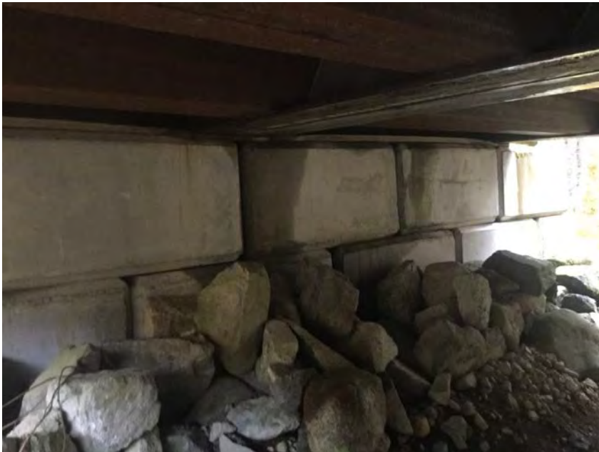
Left Bank Abutment when facing downstream
