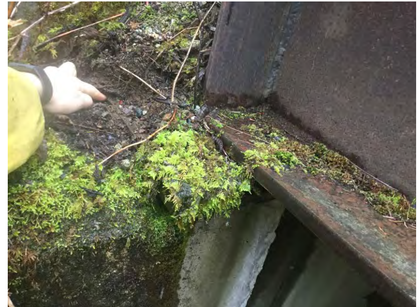
Bearing - note bearing plate note completely on lock block (back of plate indicated on photo)
